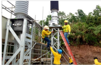
Power Plant Construction
