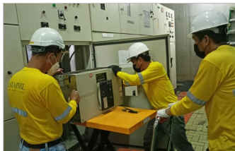
Retrofitting and Upgrades
