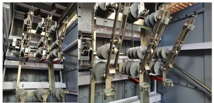
Eleron 15kV LBS with anti single phasing
