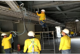
In-Plant Electrical Works
